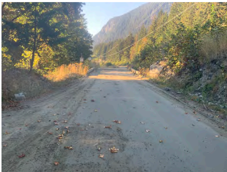
Approach from Right Bank when facing downstream
