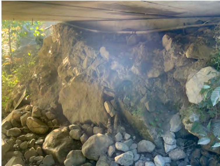
Right Bank Abutment when facing downstream
