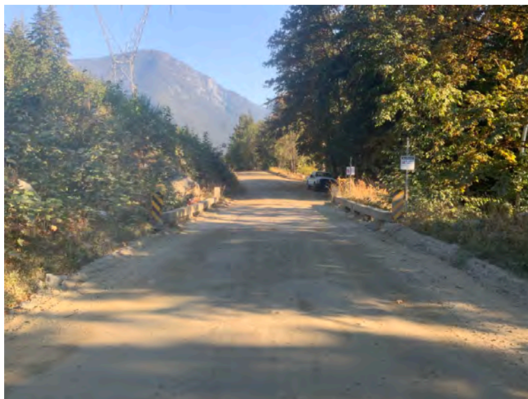
Approach from Right Bank when facing downstream
