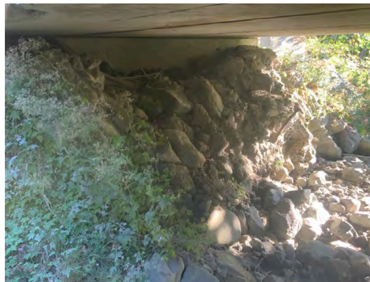
Left Bank Abutment when facing downstream
