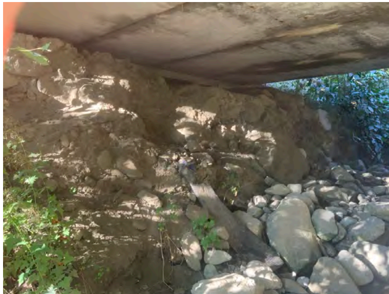
Right Bank Abutment when facing downstream
