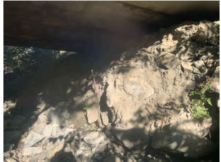
Left Bank Abutment when facing downstream
